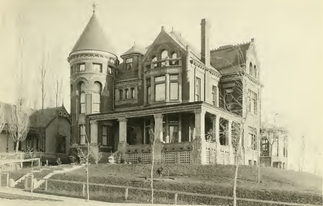
RESIDENCE OF MR. JOHN SCOWCROFT.
