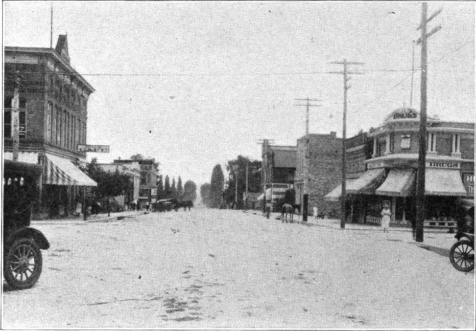
LOOKING NORTH ON MAIN STREET FROM DEPOT STREET, PAYSON
