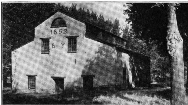
OLD MILL ERECTED BY BRIGHAM YOUNG IN 1852 AND STILL STANDING IN WHAT IS NOW LIBERTY PARK, SALT LAKE CITY
