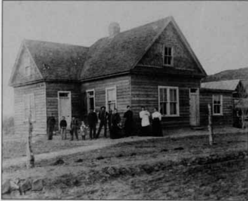
The Bradshaw Hotel in Hurricane, c. 1910. (Photograph by William L. Crawford, J. L. Crawford Collection)
