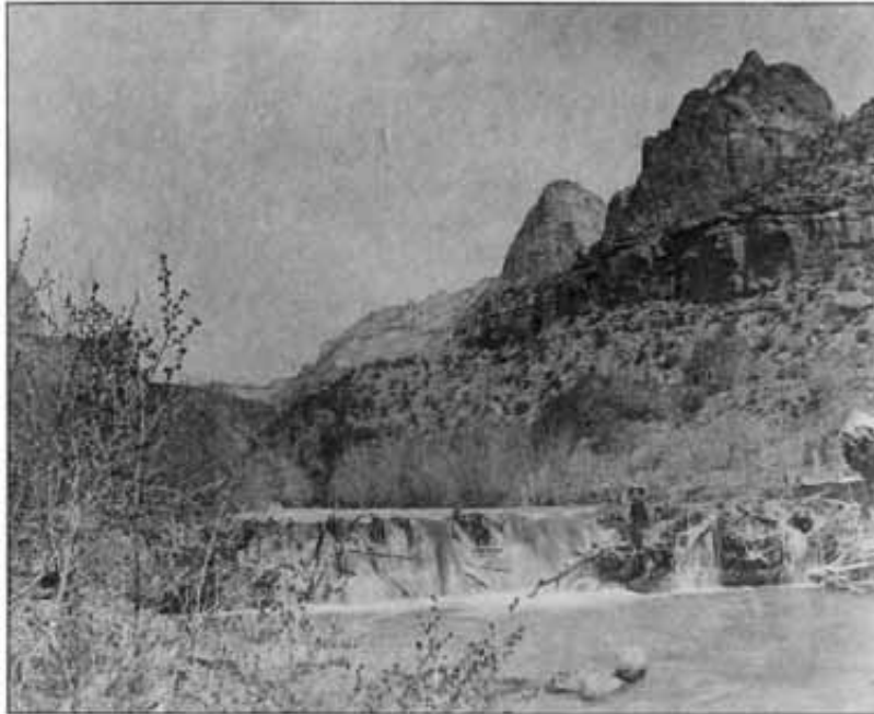
Built with trees and boulders, this dam on the Virgin River was located in what is now Zion National Park. (J. L. Crawford Collection)
