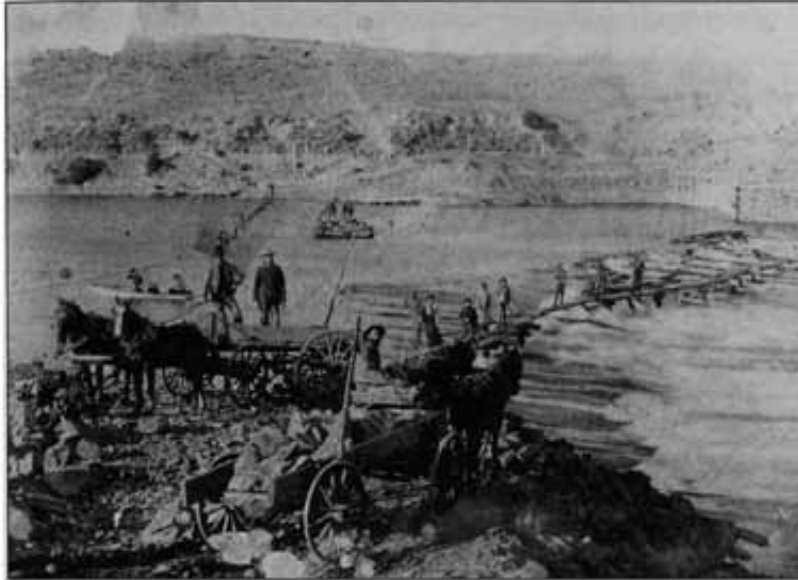
The Washington Field Dam, completed in 1891. (Lynne Clark Collection, donor—Larue Prisbrey)
