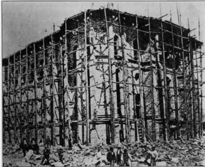
St. George Temple under construction. (Lynne Clark Collection, donor—Will Brooks)
