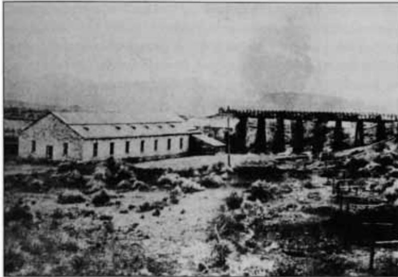
The Cotton Factory and mill race, completed in 1866. Two stories were added soon thereafter. (Cuba Lyle Collection)
