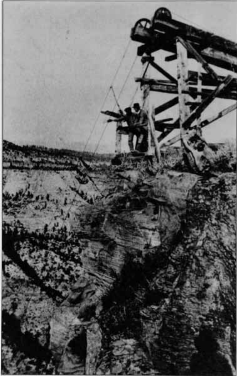
C. Y. Rozencrans and William L. Crawford standing on a platform of the upper cable frame which was built by David Flanigan between 1888 and 1901. (Photograph by Putnam & Valentine, Los Angeles, California, J. L. Crawford Collection)
