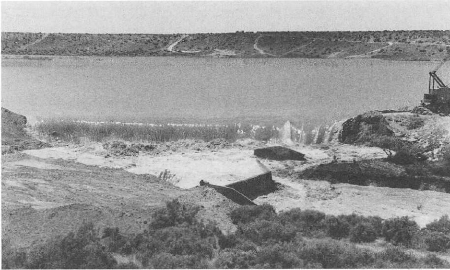
The DMAD Dam on the Sevier River northeast of Delta being washed out during the 1983 flood. (Great Basin Historical Society)
