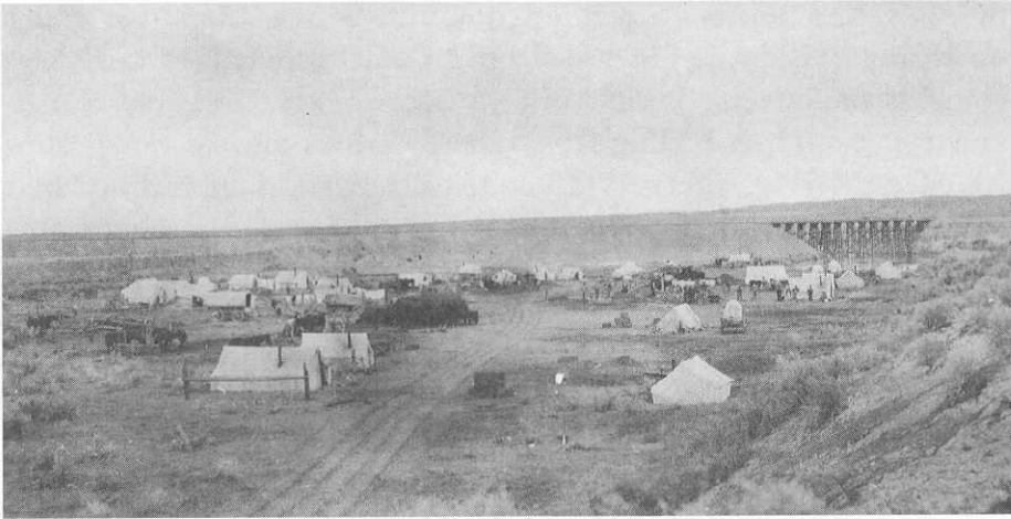
Dam construction camp north of Burtner about 1908 with railroad trestle in the background. (Utah State Historical Society)
