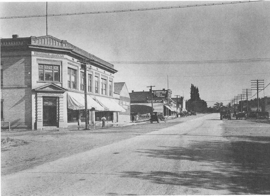
The concrete road built through Davis County can be seen running along the middle of a wide right-of-way in this August 1920 view of Kaysville's Main Street. (Utah State Historical Society)
