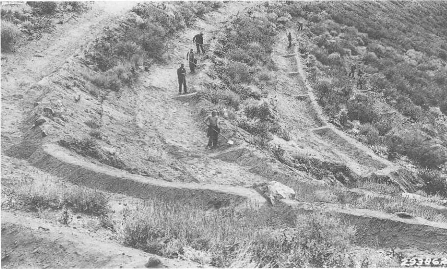
The unique terraced trench system built by Civilian Conservation Corps men on the Davis County watershed (seen here) had application in many other western American locations. (Utah State Historical Society)
