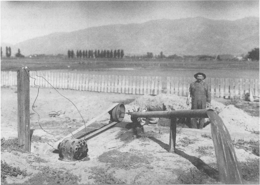
Electricity furnished by the Utah Power and Light Company allowed this Davis County farmer to pump water from an irrigation pond onto his fields in 1913. (Utah State Historical Society)
