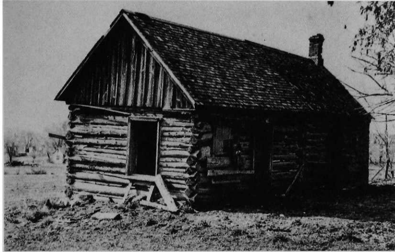
Double Log house with shingle roof, Richmond, 1870s. (Special Collections Merrill Library, USU)
