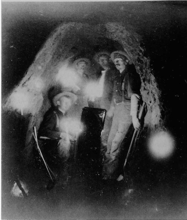
Miners working inside Sundown Mine, La Plata, 1892. (Special Collections Merrill Library, USU)
