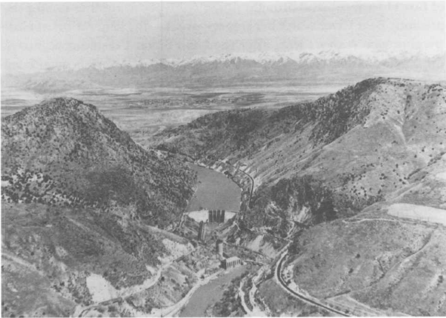
View of Bear River Canyon with the Cutler Power Plant, reservoir, dam, pipeline, surge tank, east and west canals, and the railroad. (Box Elder County)
