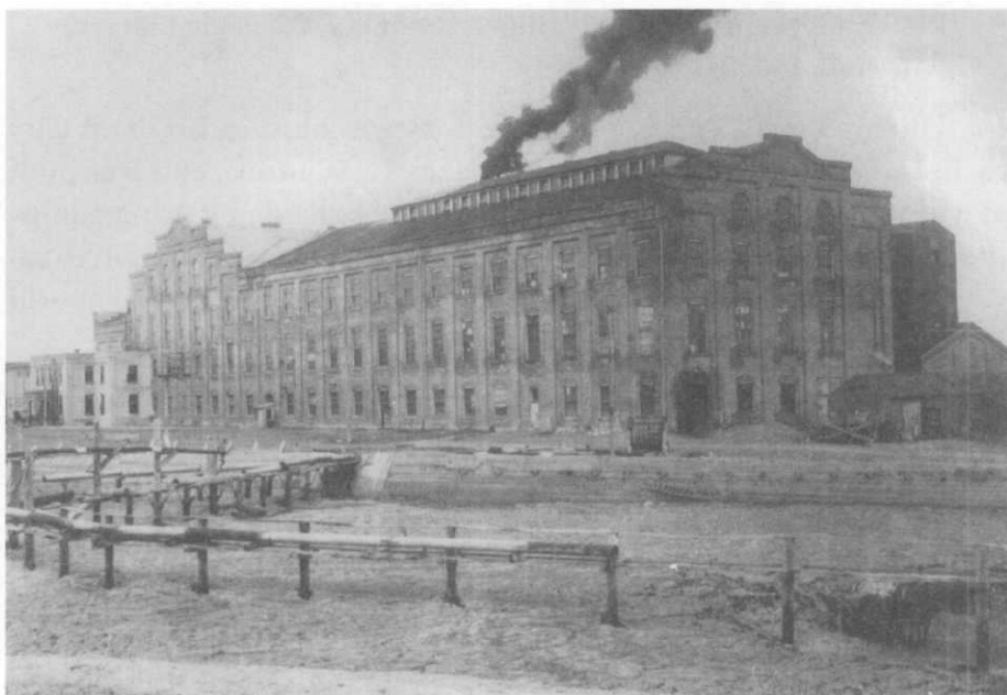
The Brigham City Sugar Factory was built in 1916 and operated until 1937. It was demolished in 1944. (Box Elder County)
