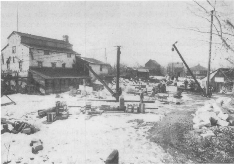
Bott's Monument in 1920. The original building was the Lorenzo Snow flour mill built in 1855–56. (Box Elder County)
