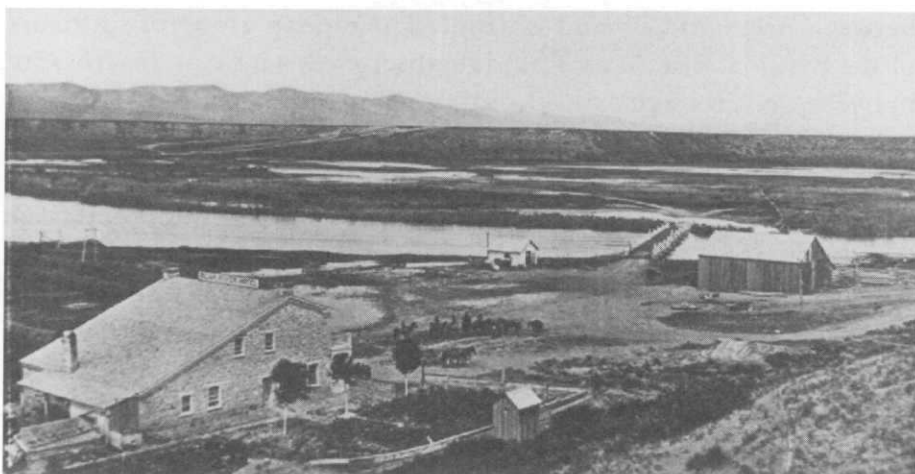
This photograph of the Hampton Stage Stop and bridge across the Bear River at Collinston was taken by W. H. Jackson in 1872. (Box Elder County)
