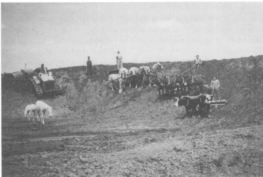
Smoothing out a stock pond site on the Adams ranch in 1939 using a caterpillar tractor, four horse fresno, four mule fresno, and a bucket scraper pulled by two oxen. (Box Elder County)
