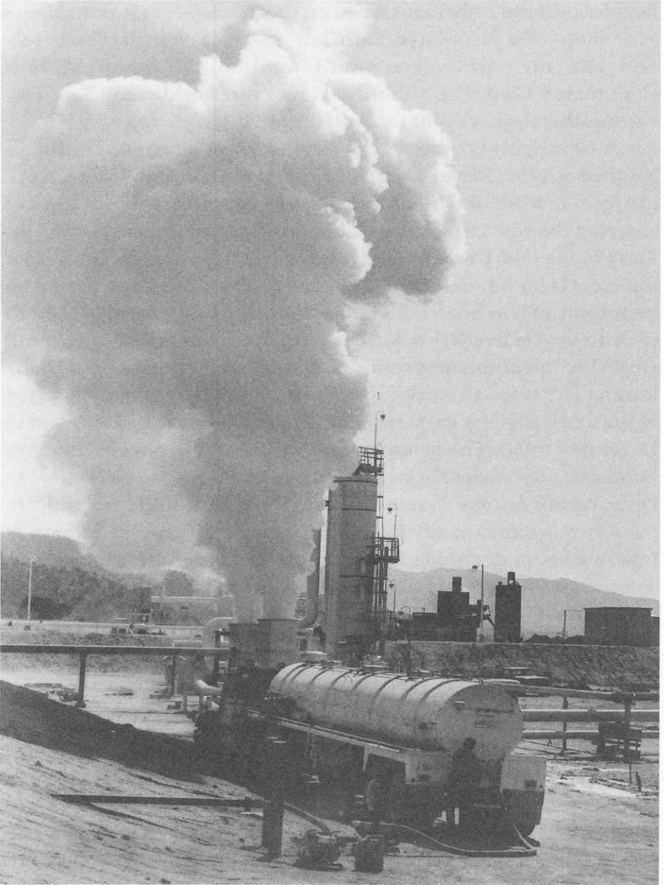
Geothermal power plant at Roosevelt Hot Springs northeast of Milford. (Courtesy Gladys Whittaker)
