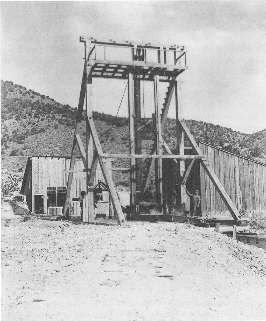
This headframe stands over a mine shaft at Newhouse. (Utah State Historical Society)
