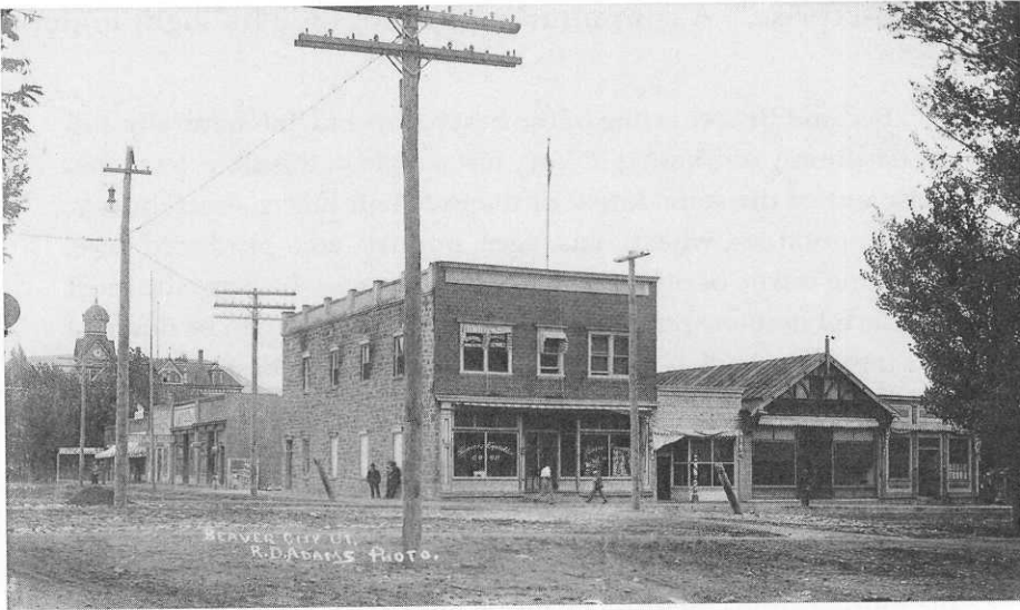
The southeast corner of Main and Center Streets in Beaver with the Equitable Co-op Building on the corner and the tower of the Beaver County Courthouse in the background. (Utah State Historical Society)
