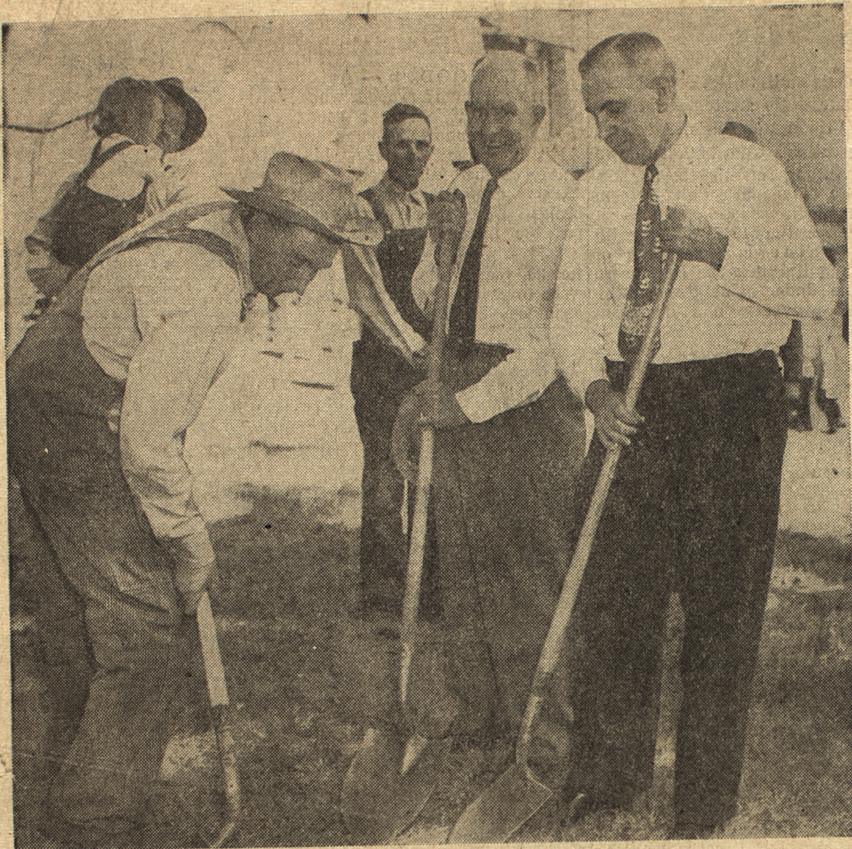
LIBERTY WARD GROUNDBREAKING —Bishop Lysle Chard of the Liberty Ward turns the first shovel of dirt for their new chapel addition. Waiting their turns are James Martin, center, member of the Ogden Stake High Council, and Arias Belnap, a member of the stake presidency. Groundbreaking was Monday evening.
