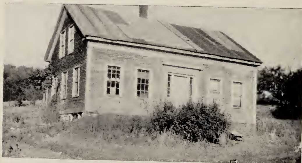
THE GAMALIEL WALDO HOUSE Middletown Springs, Vermont
