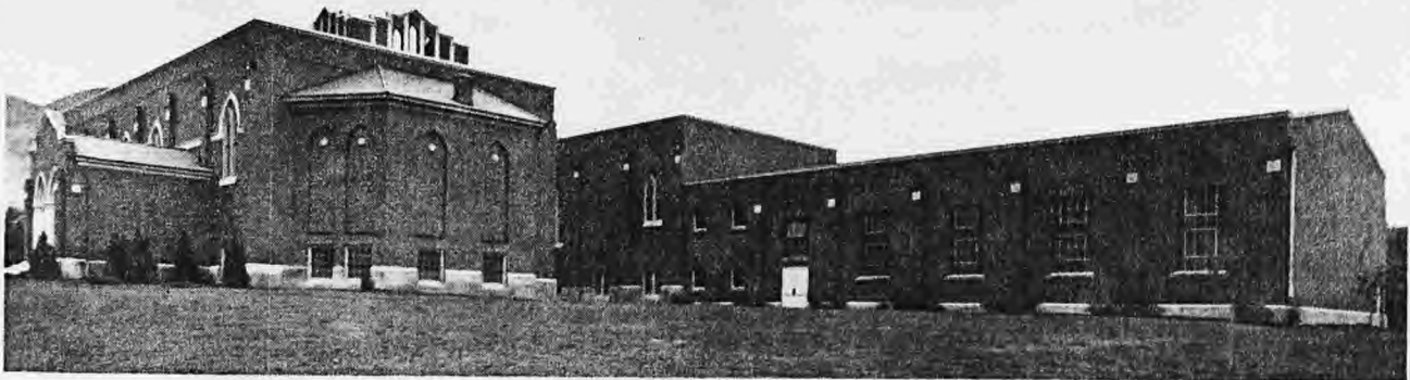
A sidelong rear view of the structure, showing the gym extension
