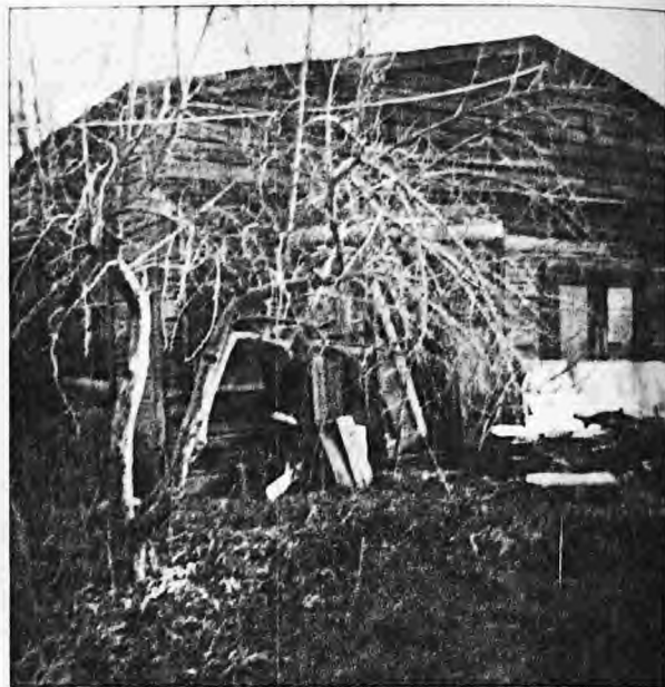
The old building that was the Minnoch Art Glass Shop (Front View) 451 30th St. Ogden, Utah
