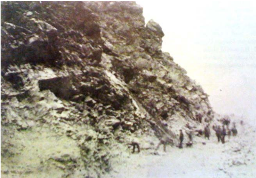
Crews hand digging a canal in Weber Canyon
