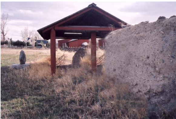
Part of the remaining mud wall which surrounded the fort
