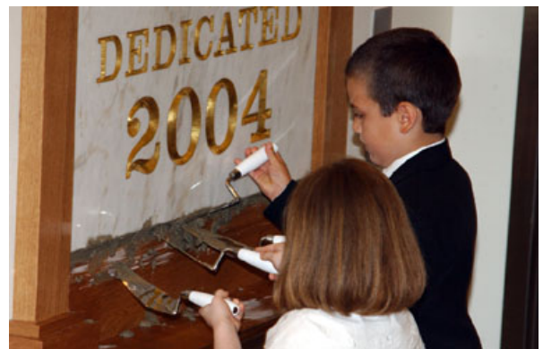
Christopher Belnap, age 7, son of Brent and Lorinda Belnap placing mortar on the Manhattan Temple cornerstone
