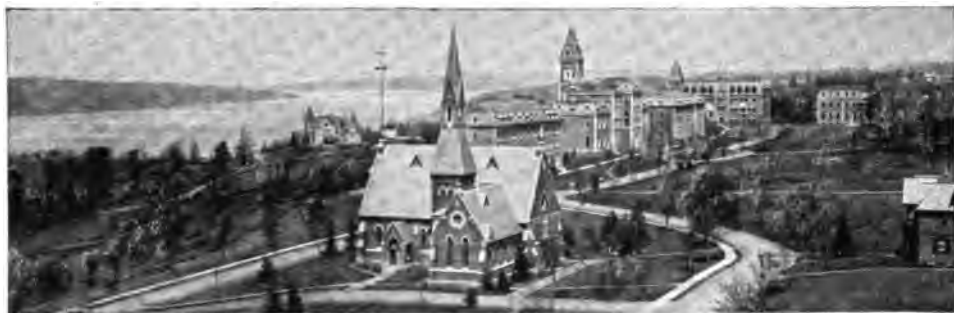
Cayuga Lake. Fiske House. Sage Chapel. Morrill Hall. McGraw Hall. White Hall. Physical Laboratory. Sibley College. General View of earlier buildings of Cornell University, from Sage College.
