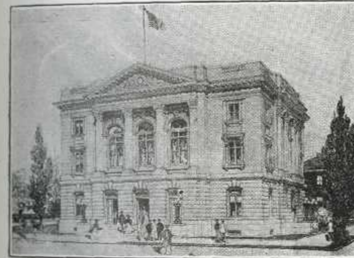
FEDERAL BUILDING, OGDEN, UTAH
